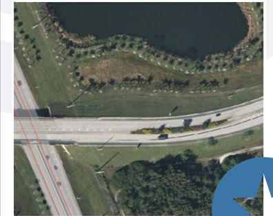
Becker Road Water and Wastewater Improvement Project
