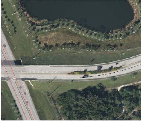
Becker Road Water and Sewer Improvement Project
