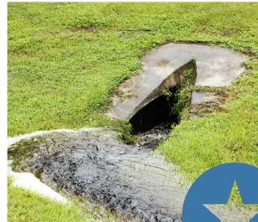
Culvert and Swale Improvements
