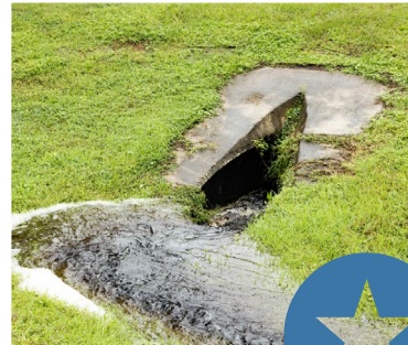
Culvert and Swale Improvements
