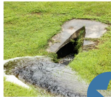
Culvert and Swale Improvements
