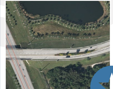
Becker Road Water and Wastewater Improvement Project
