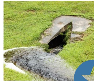
Culvert and Swale Improvements
