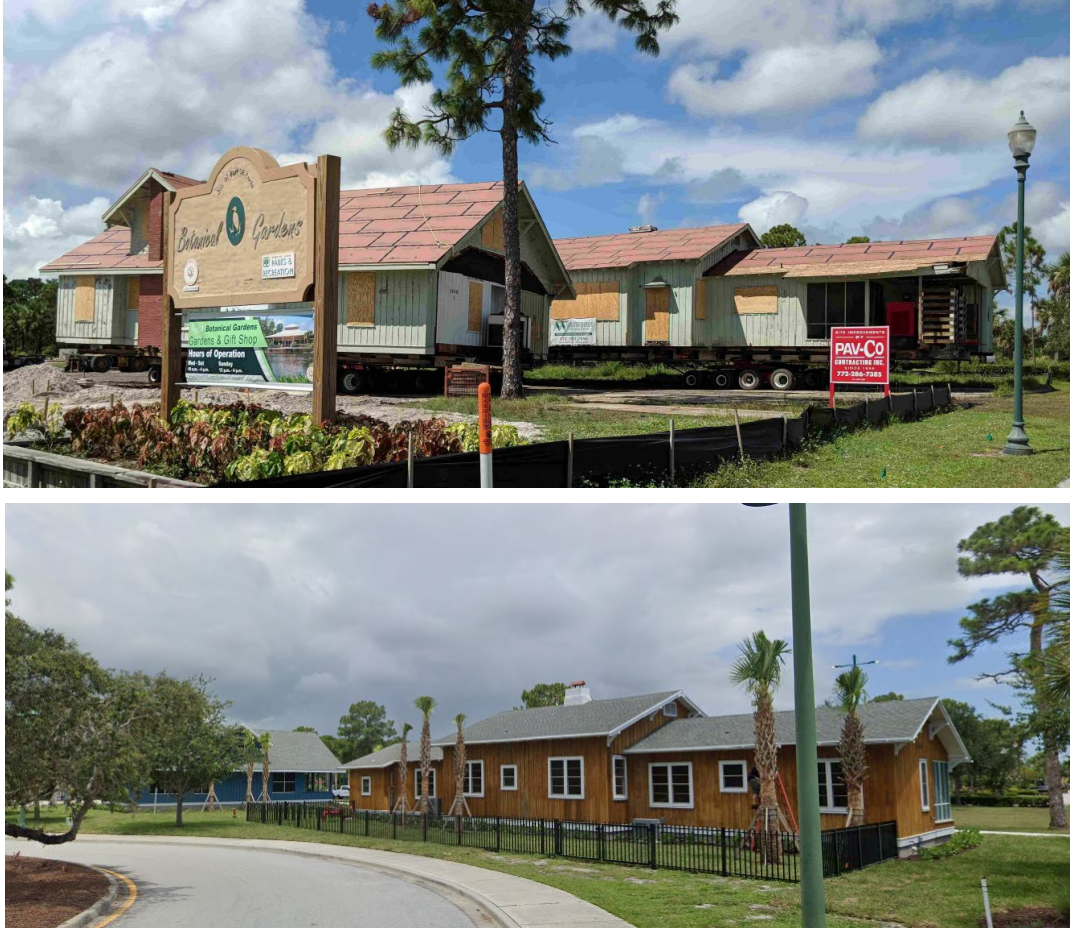
Figure 3 - 6. Peacock Houses (before and after relocation and renovation)
