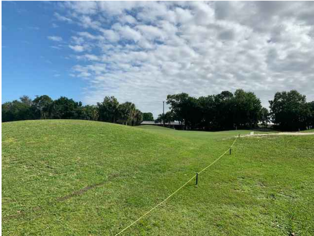
View 1 of Monopine Tower Location Before Installation. (Looking East)
