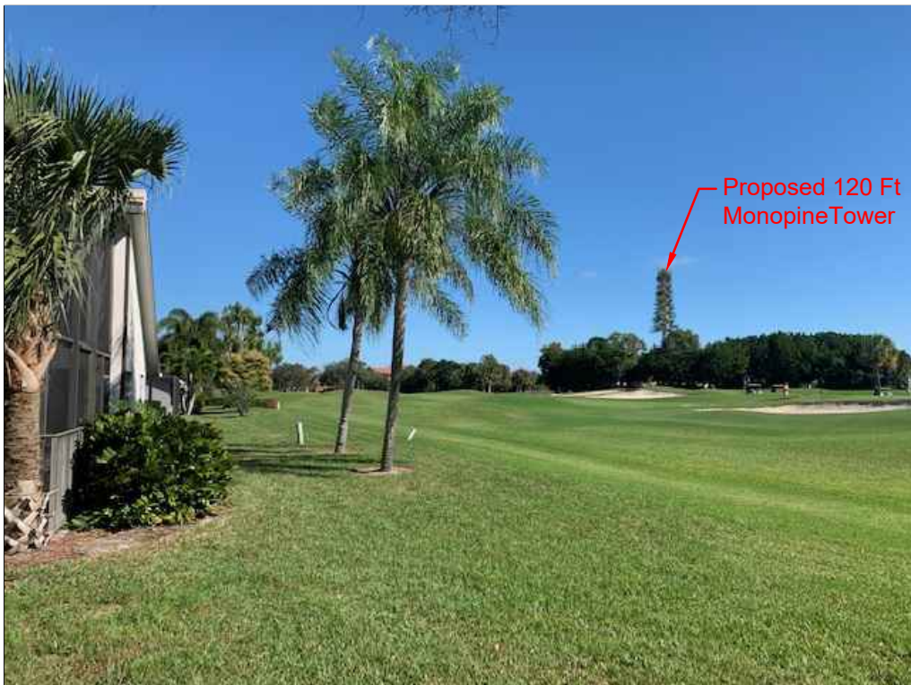
View 2 of Monopine Tower Location After Installation. (Looking North East)
