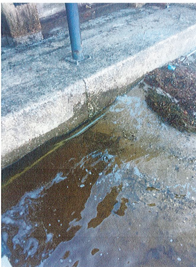
Fresh water side with typical cracks 1/16" wide. Also the cable for the cathodic protection has re-surfaced.
