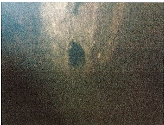
Two holes in the sheet pile
