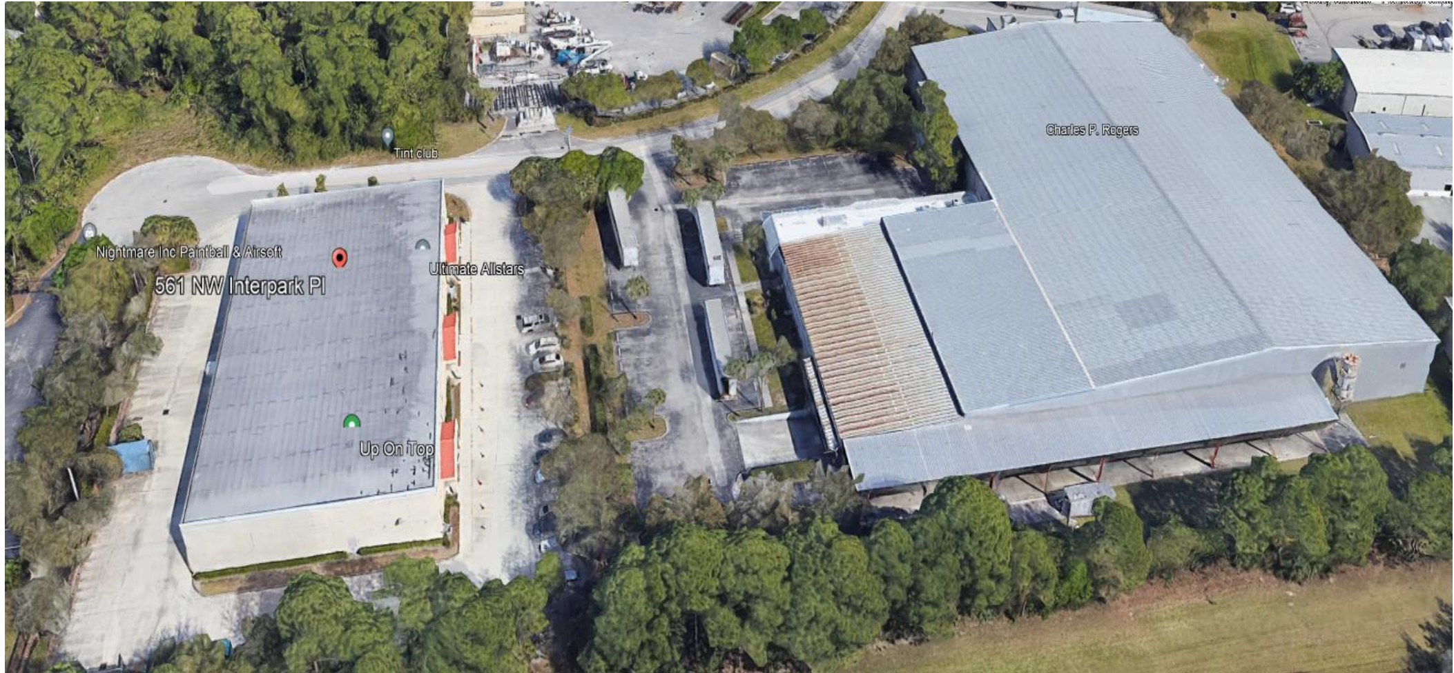
Aerial Site View
