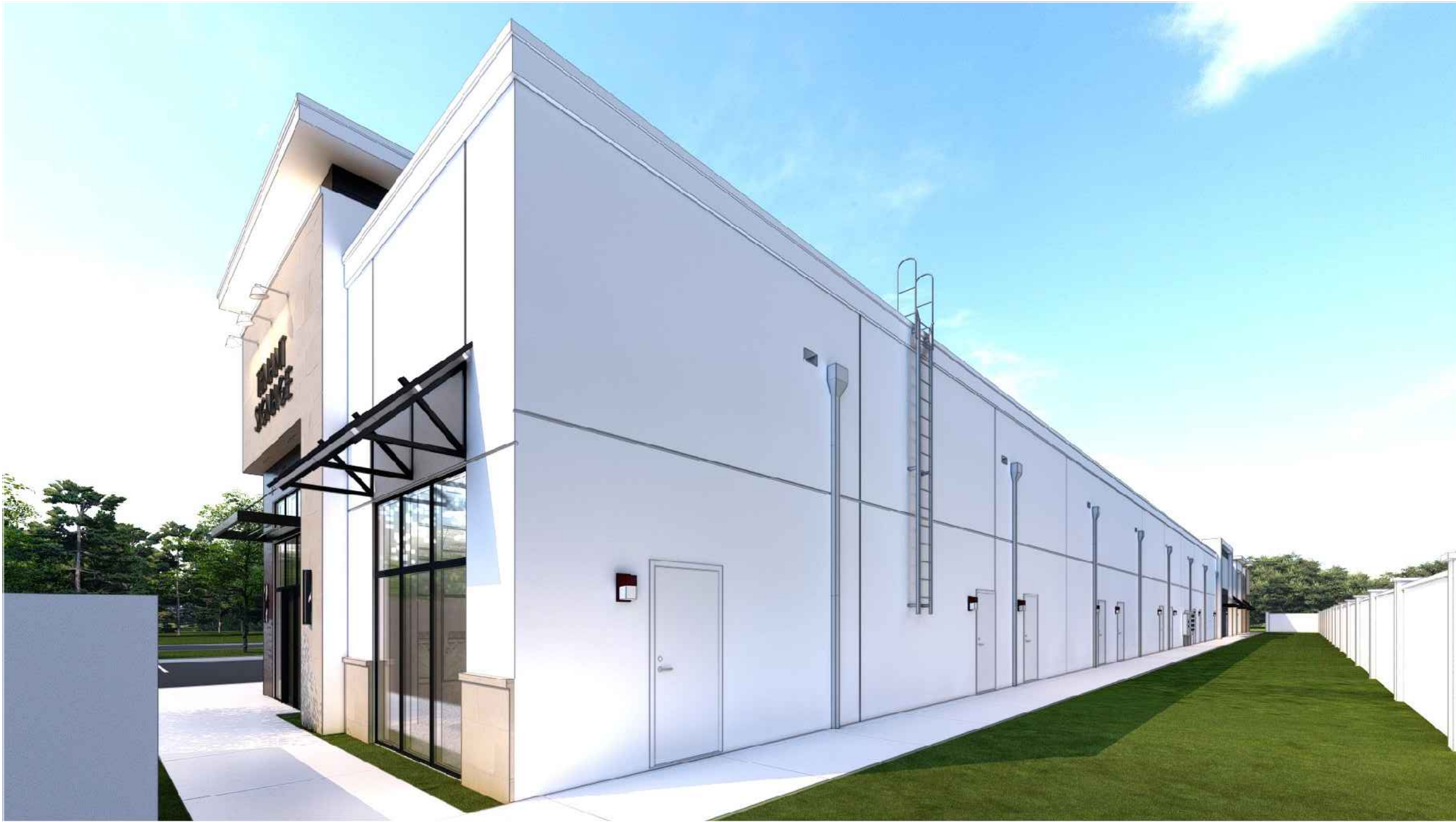
REAR ELEVATION - PARKING LOT
